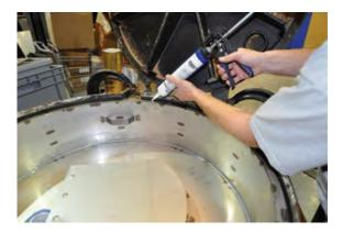
3. Put a bead of silicone around the top flange of the manhole scrubber. Ensure a positive seal to f orce all gases though the media canister chamber.
