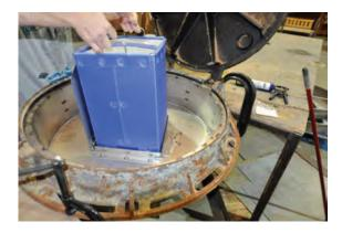
5. Insert media canister (PART # OCI-2050-50) by the handles into the media canister chamber. Push down the canister by its handles until completely in. Close hatch door ensuring it is completely closed before installing manhole lid.
