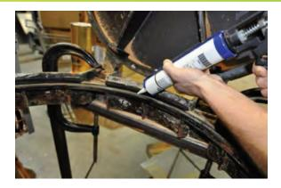
1. Put a bead of silicone on the interior ring of manhole cover frame.
