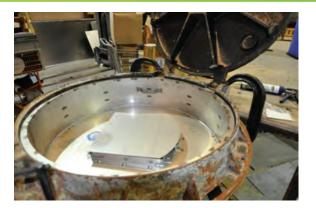
2. Lift empty manhole scrubber by the provided handles, and lower the unit into the manhole opening.
